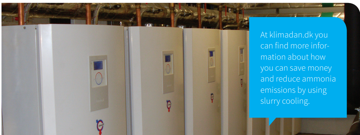
Cascade heat pumps are at the heart of a slurry cooling system
